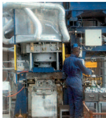
The forging installation
