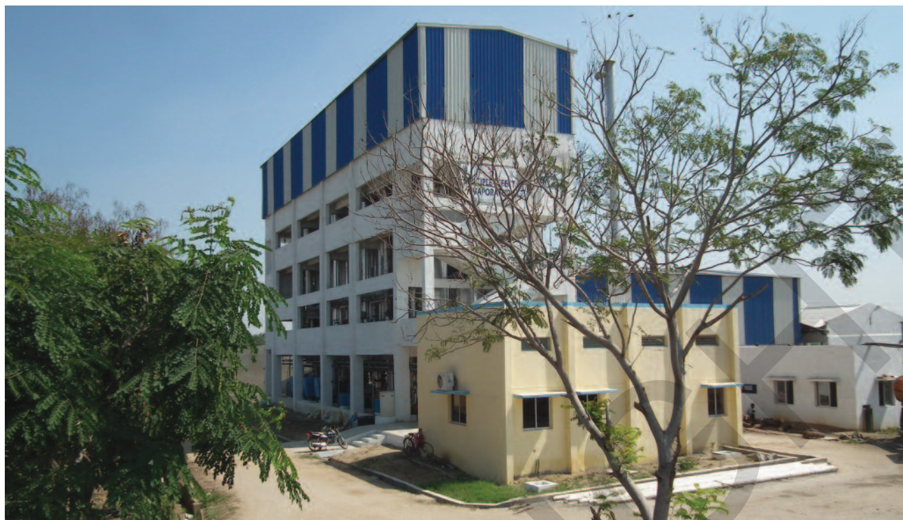
CETP plant, Ranipet. ALL IMAGES: WTP
